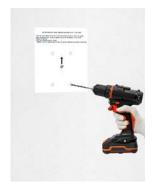
Drill (x4) 8mm holes 2 inches deep using the mounting template.
